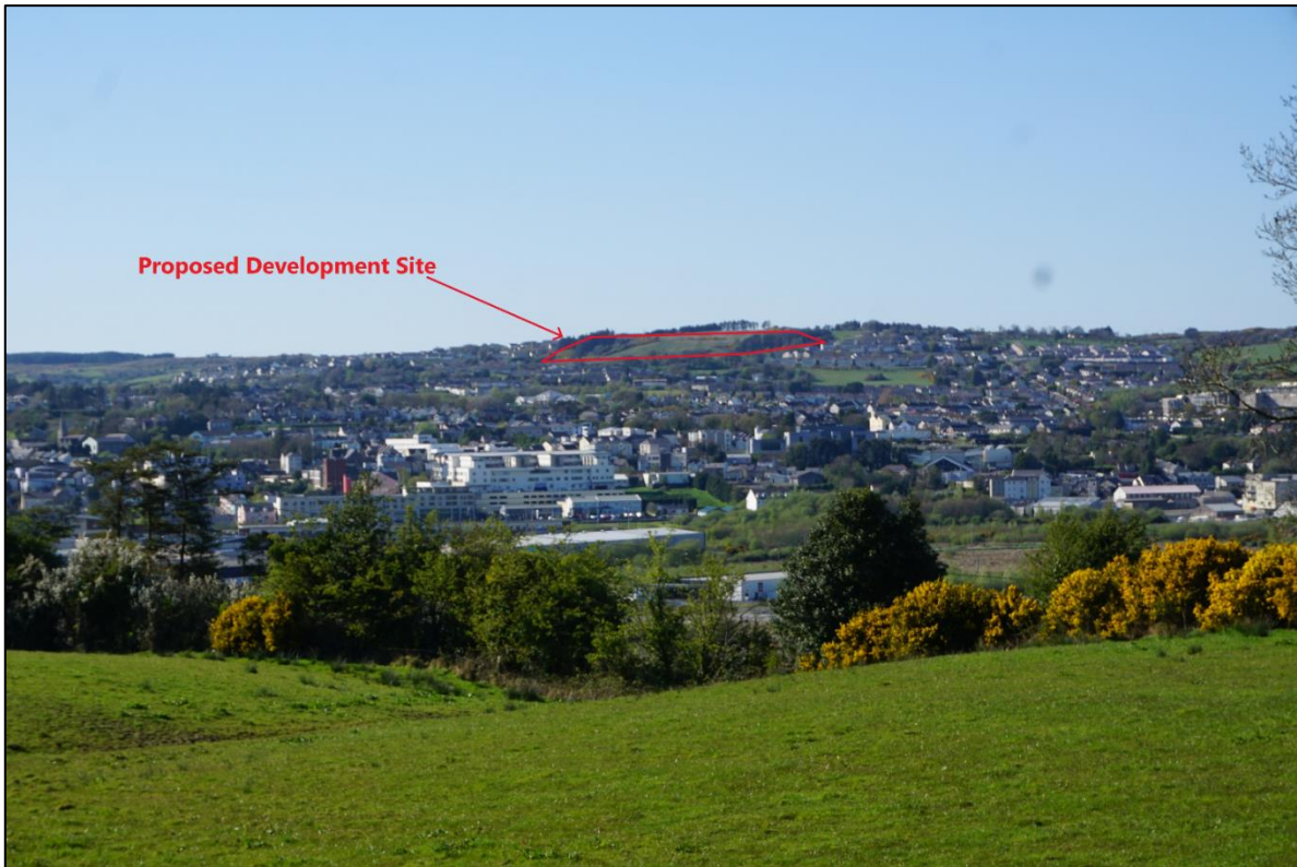
GPS -7.7155, 54.9412 Distance to site: 3.34 km Elevation: 52m Direction of view: NW Description: Application site visible as part of the view of Letterkenny town on approach to Letterkenny on an elevated section of the L-1114 from the south.
